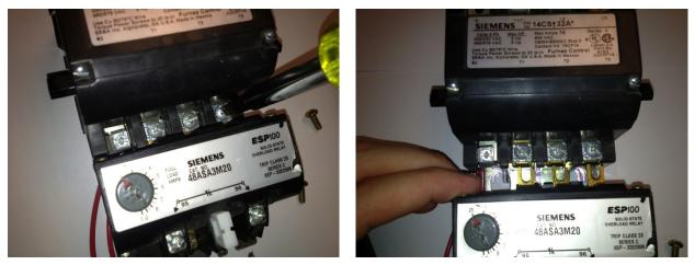
5. Remove the old **ESP100** overload and place the new **ESP200** overload on the back board.
