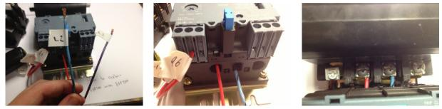
10. Remove the label and feed the load wire (L3) through the right hole in the ESP200. Terminate this wire onto the T3 terminal on the contactor.
