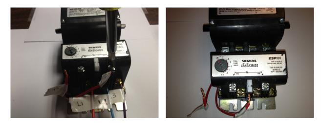
3. Remove the two bronze screws holding the ESP100 to the back plate.
