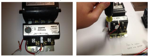
4. Loosen the load screws on the contactor and slide the ESP100 off.
